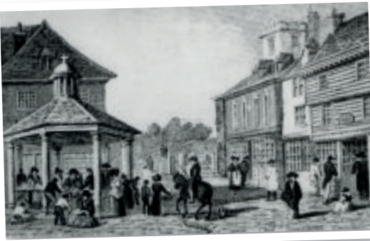
The new market house after the old one was demolished in 1809
